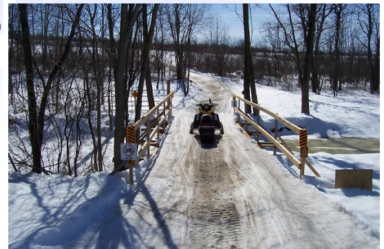
Knox Ball Field Bridge - March 10, 2010
